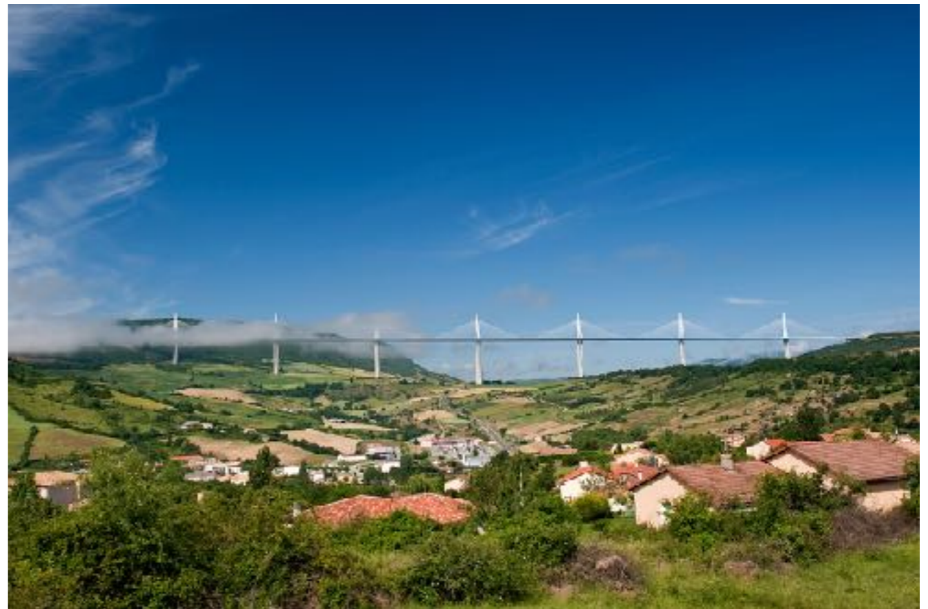
Millau Bridge: engineer Michel Virlogeux, architect Norman Foster
