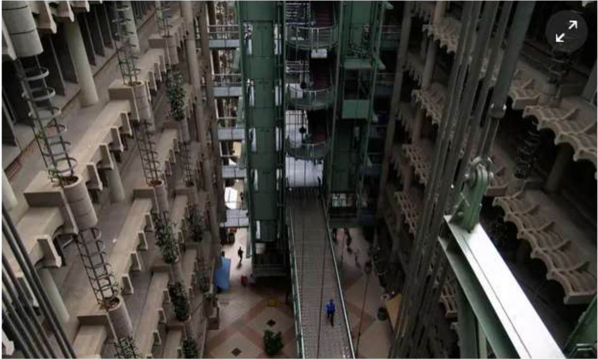
▲ The Eastgate building in Harare has no air-conditioning or heating, yet stays regulated all year round using a design inspired by indigenous Zimbabwean masonry and termite mounds. Photograph: Ken Wilson-Max/Alamy
