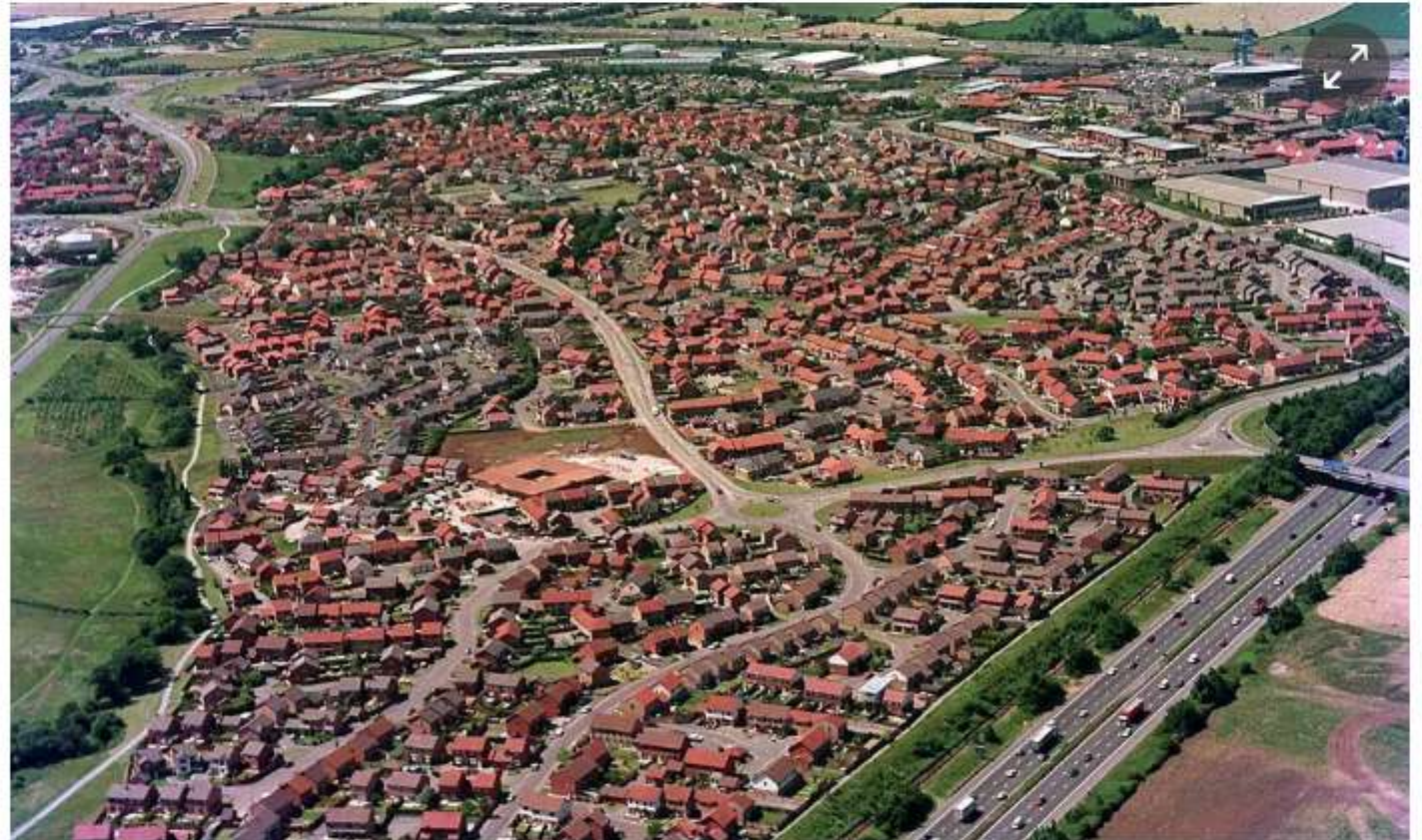
▲ Bradley Stoke, Bristol, an example of the late 20th-century housing estates that followed rules set out in 1977's Design Bulletin 32. Photograph: SWNS
