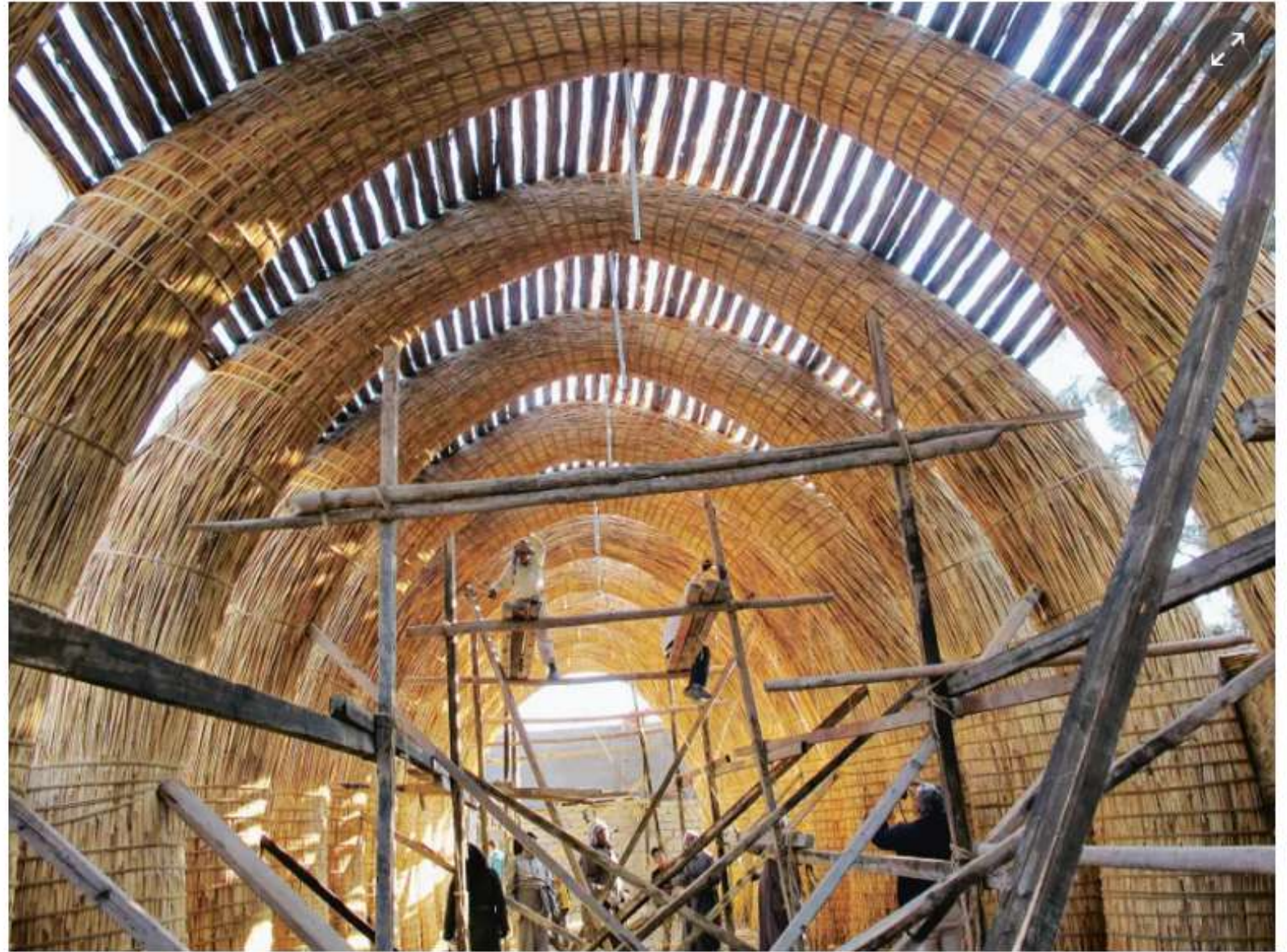
▲ An entire Ma'dan house, known as a mudhif , is built entirely of qasab reed
