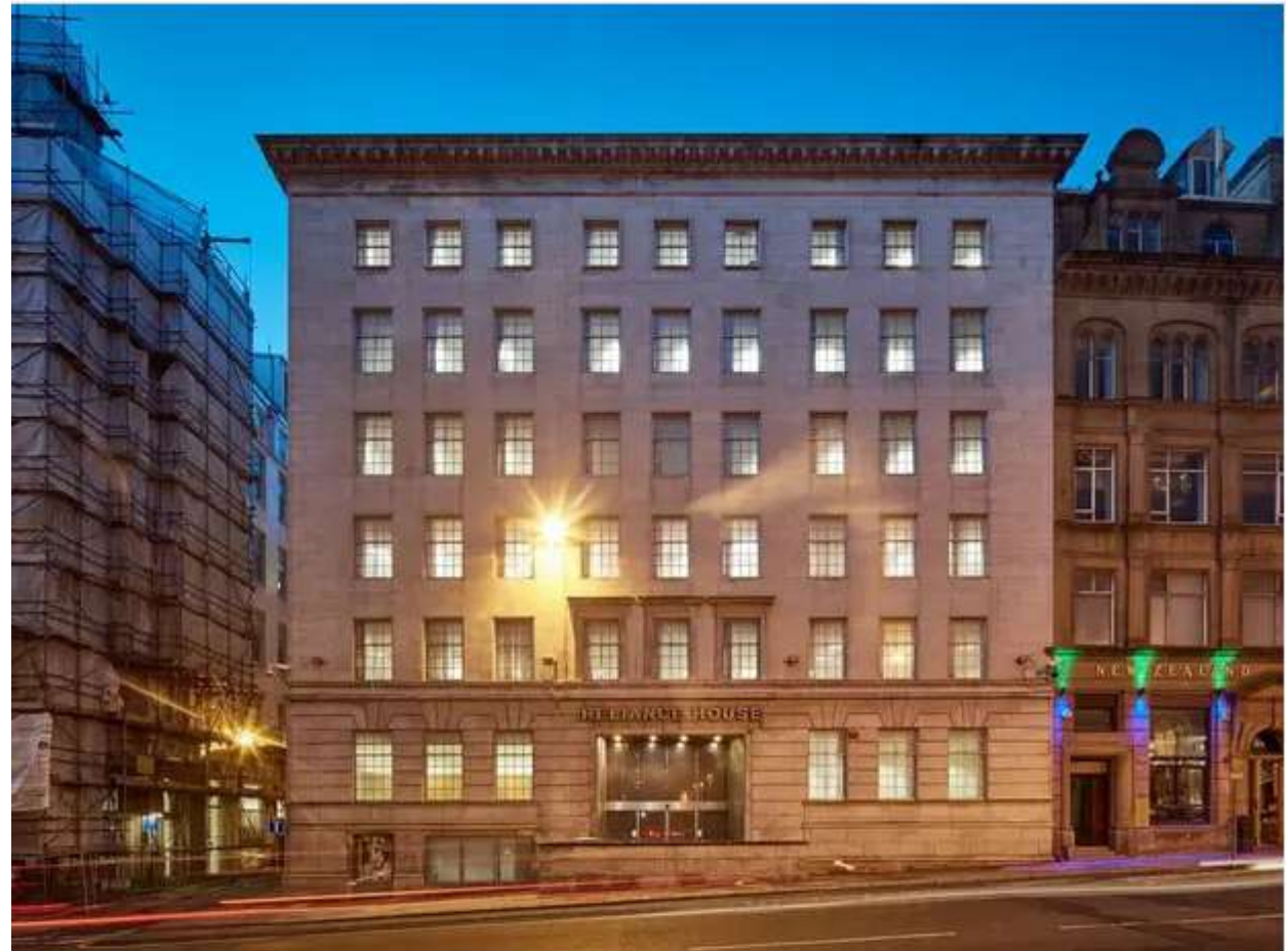
▲ Reliance House, Liverpool, a £24m project. Five of the basement flats have no windows. Photograph: © 2016 Reliance House
