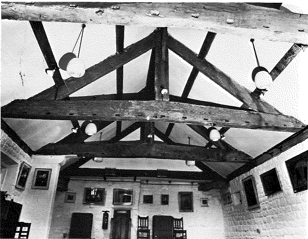
The 17th century king post roof.
