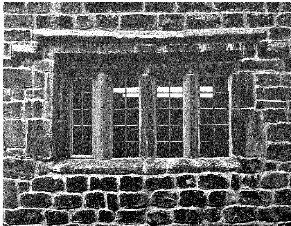
The mullioned windows with drip-mouldings.
