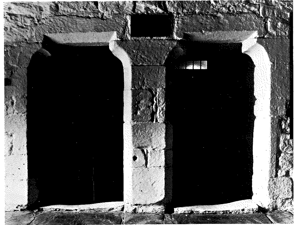
The Caernarvon arches in the screens passage.
