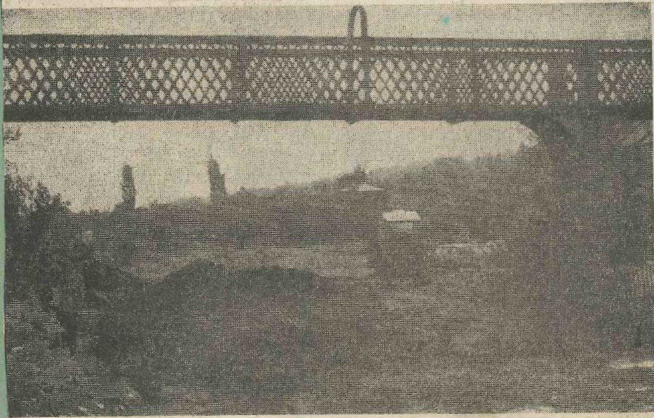
Another major development was the start of work on a new Hillards superstore on the old railway goods yard at Springs Lane, following the company's successful appeal against refusal of planning permission.
