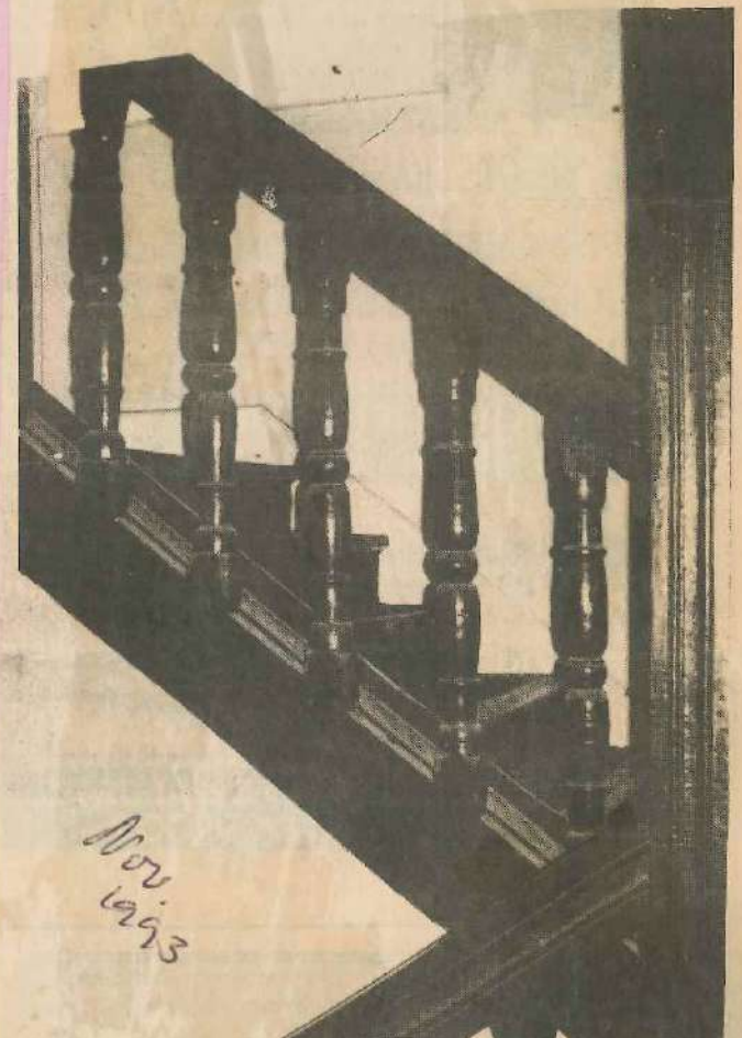
Part of the staircase of 1620
