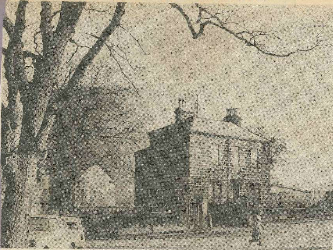
Property in Lower Wellington Road, Ilkley, which once housed the Manager of Ilkley Gas Works in the days when gas was manufactured on the site is another link with the past which is shortly to disappear. The property is to be demolished.
