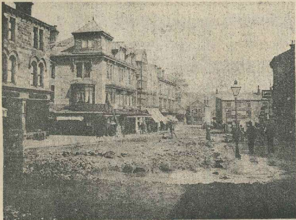
The scene in Brook Street after the bursting of the culvert. Water flowed from here to the Star, Wharfedale and Wheatshaf Inns at the bottom causing a considerable amount of damage.
