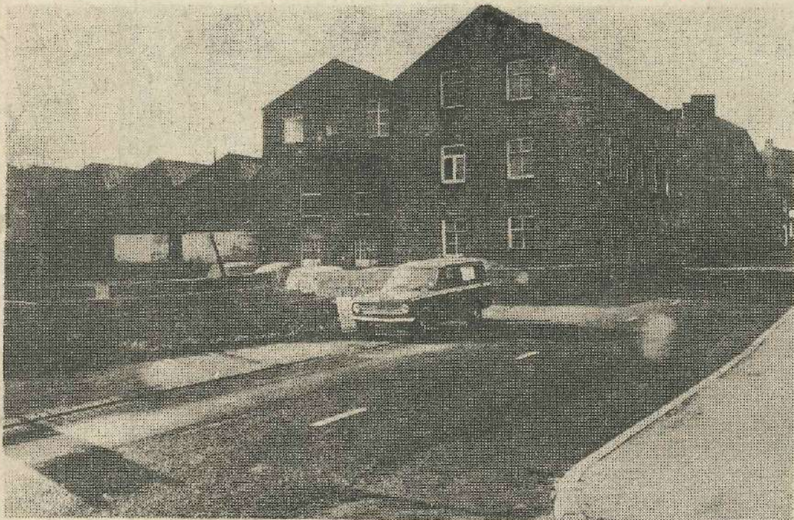
A suggestion that one of Addingham's old mills known as the Wolsey Shed off Main Street, should be demolished (subject to the owners' contribution) under a special environmental improvement scheme is to be investigated by Skipton Rural District Council. The photograph illustrates the premises looking towards the west with Main Street in the foreground.
