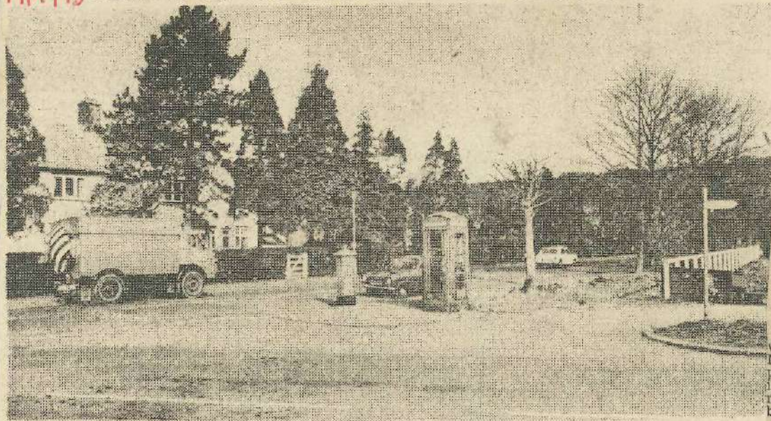
Improving the sight-lines at the Cricket field corner of Middleton Avenue, some of the trees have been removed and the old entrance changed leaving the telephone kiosk and the old fashioned pillar box on an island site.
