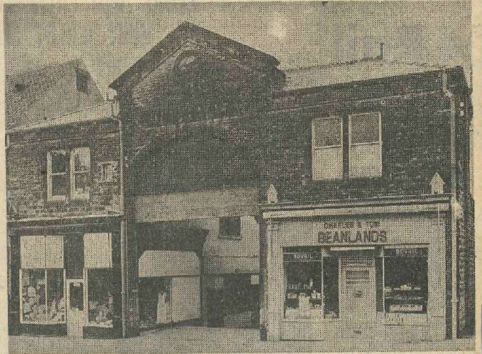
Planning permission has been granted by Bradford District Council's Development Control Panel for alterations and renovations to the old arcade at South Hawskworth Street, Ilkley, which is pictured above.
