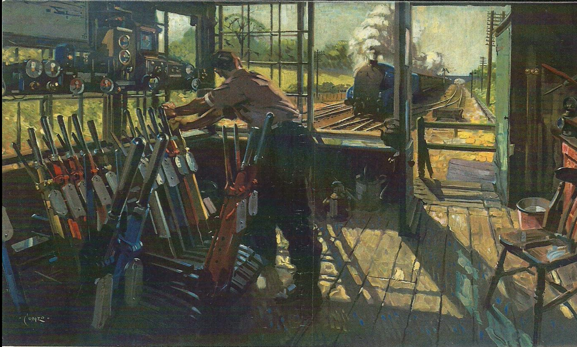
GREENWOOD SIGNAL BOX, NEW BARNET
