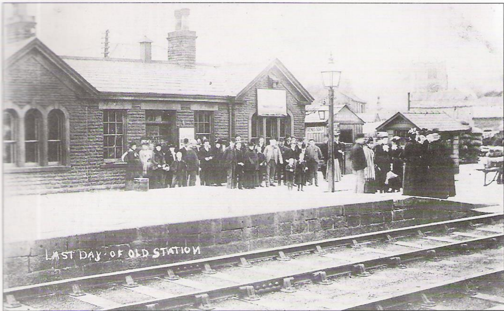
The Keighley bound platform at the old railway station. Note the Parish Church tower in the background.
