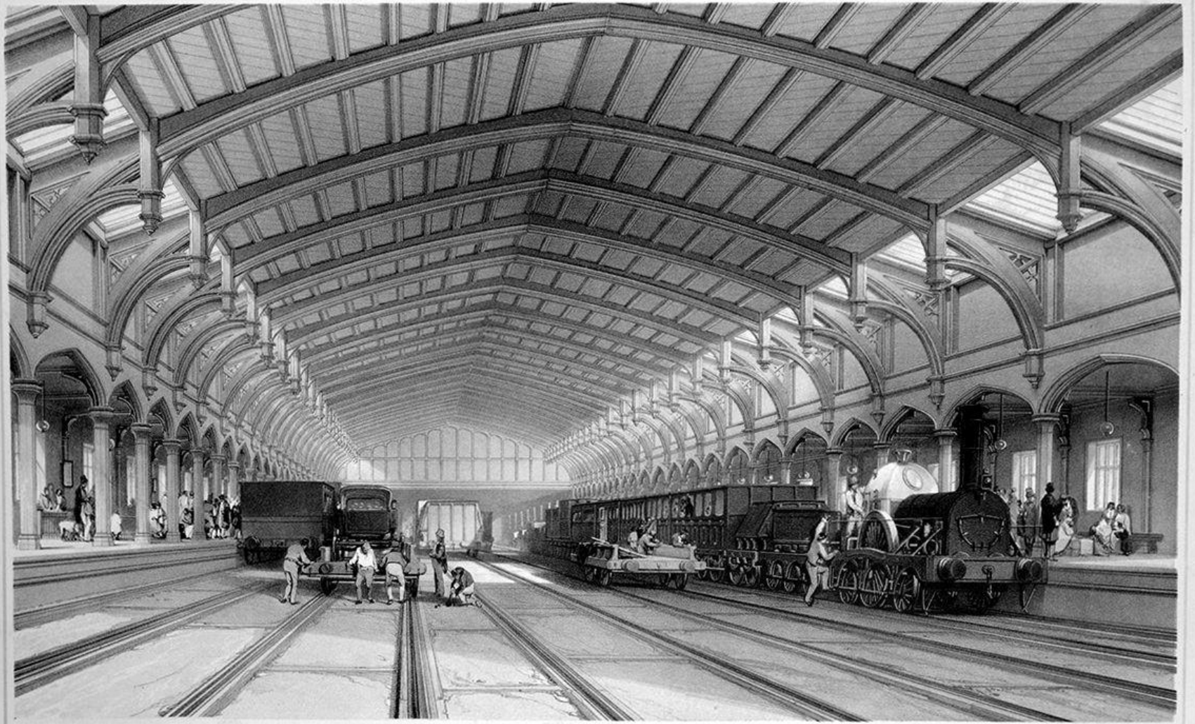
Architectural drawing of the interior of the Great Hall, London, by J. C. Ince.
