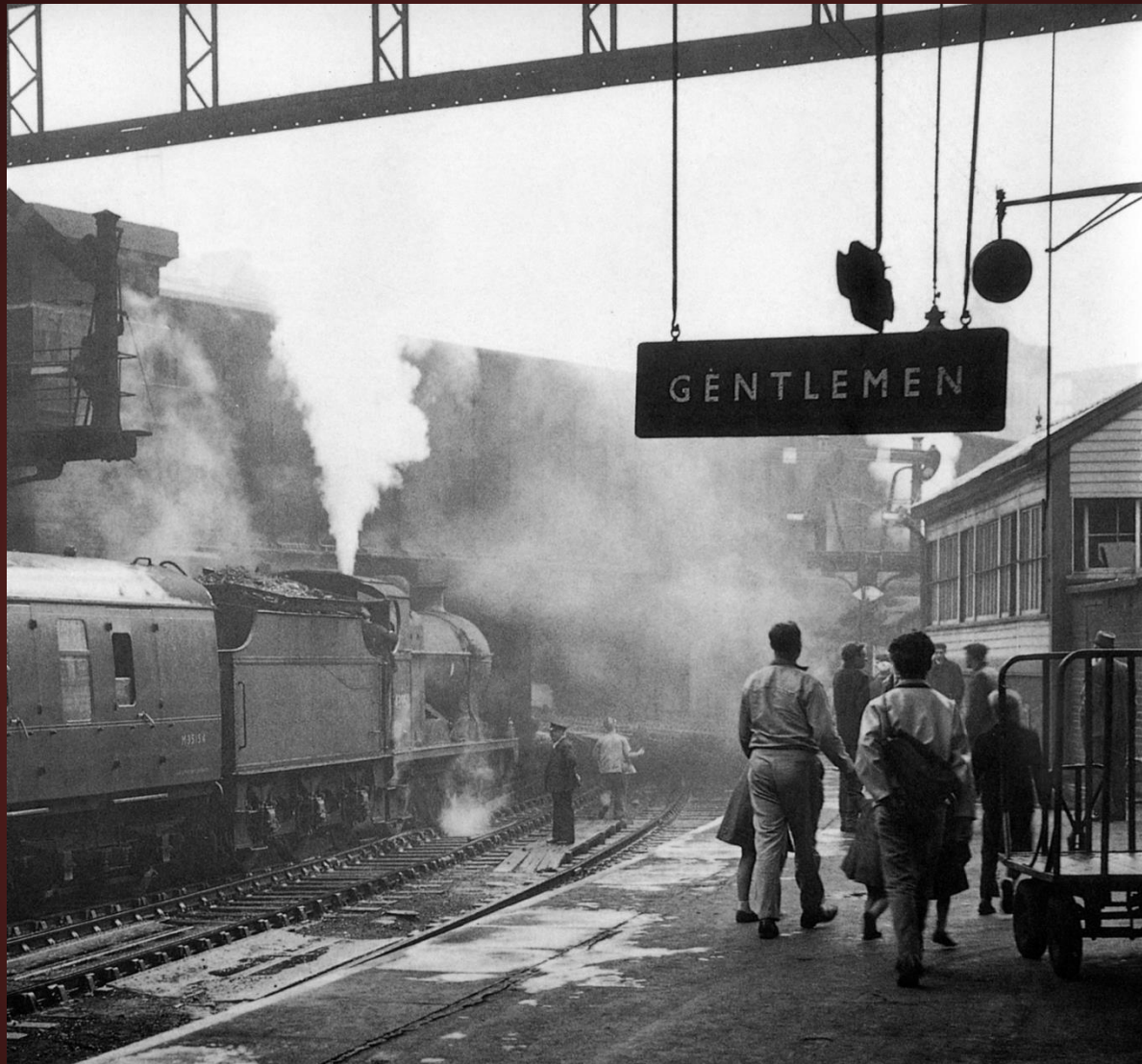
Replacement for failed 'Peak' on up Devonian
