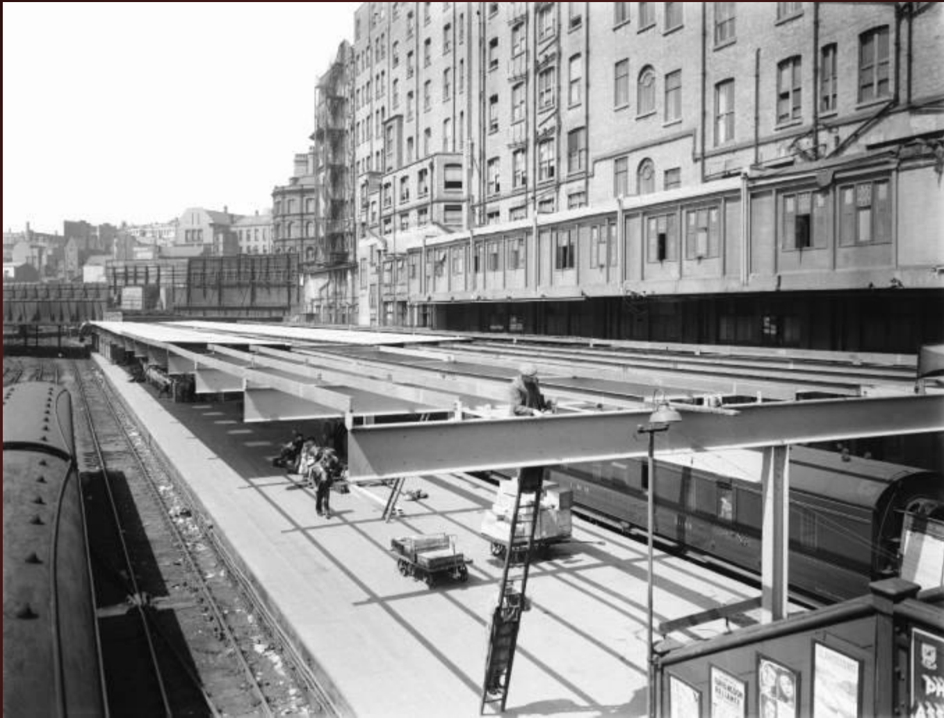
Rebuilding LNW side, 1947
